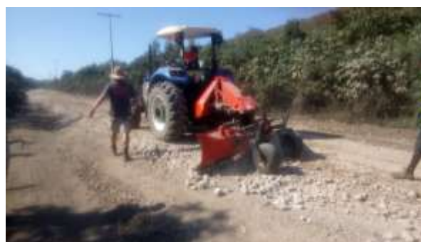
Image 18: Spreading the gravel
