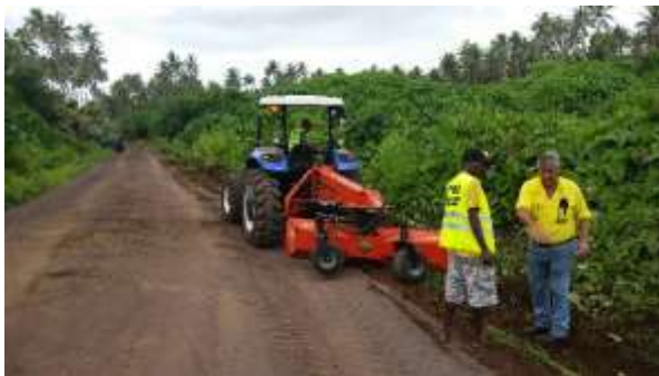
Image 7: Training of the operators on Ambae (grading)
