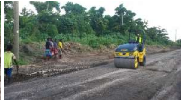
Image 22: Compaction with combi-roller
