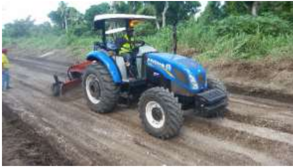
Image 21: Shaping the camber
