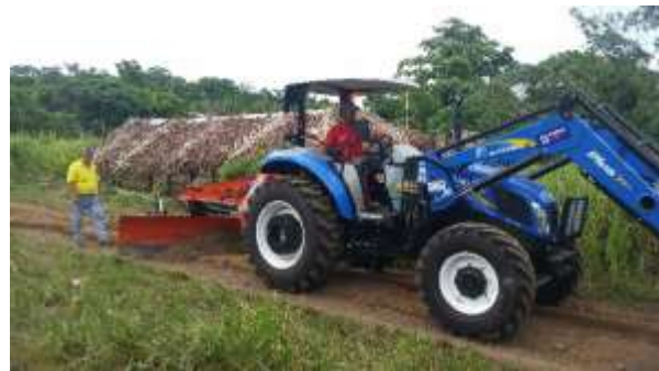
Image 8: Training of the operators on Ambae (grading)
