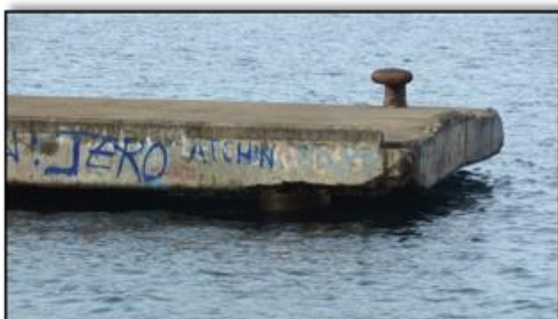
Figure 55 Wharf with low freeboard at high tide
