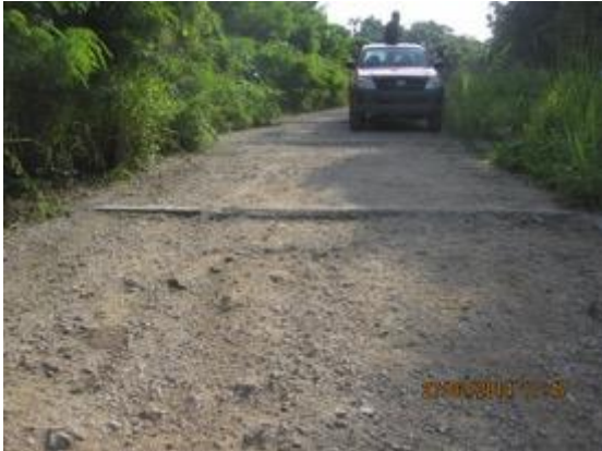
Figure 38 Horizontal scour checks
