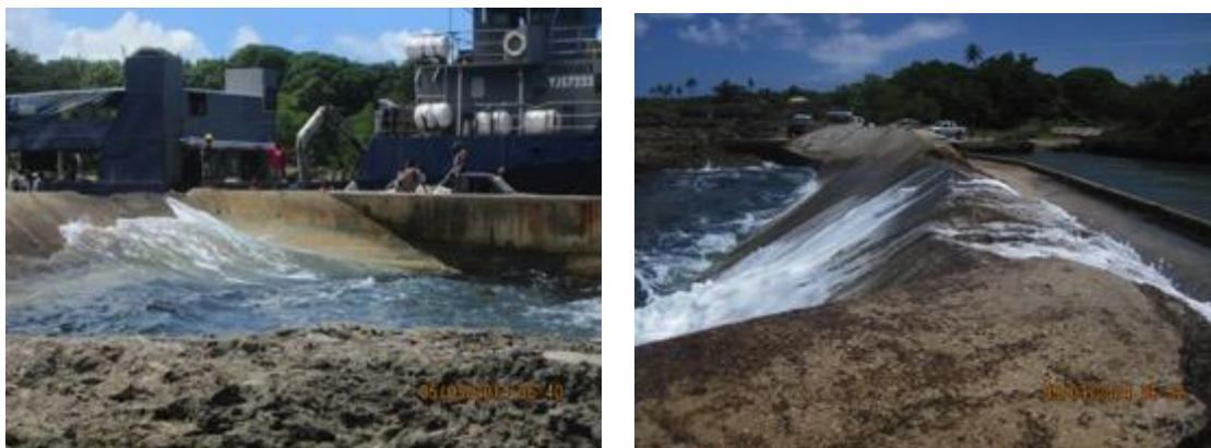
Figure 54 Wave run up and over topping
