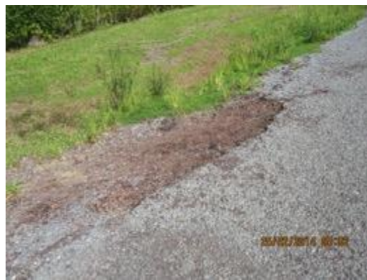
Figure 14 Pavement and shoulder breaking up on Efate and Ambae roads
