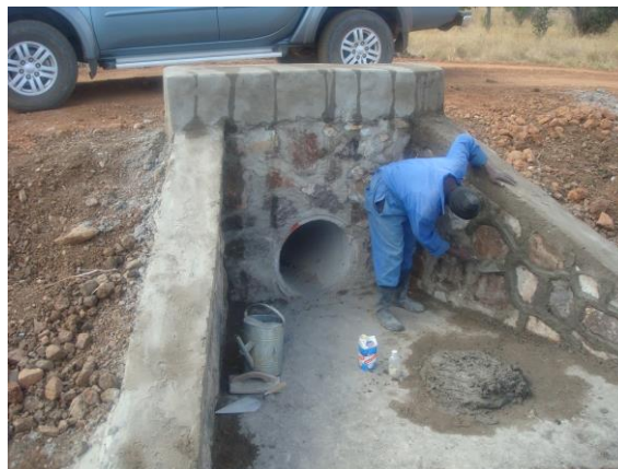
Figure 29 Stone masonry works
