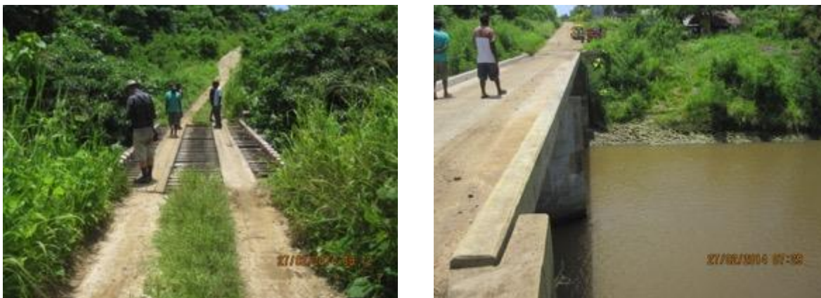
Figure 31 Wooden bridge and concrete bridge, Malekula
