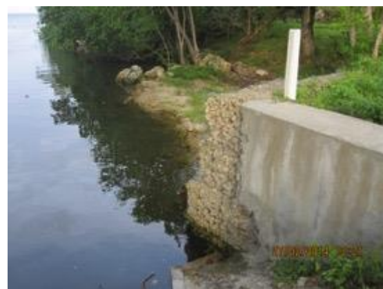
Figure 34 Gabions used in water crossings (Malakula)
