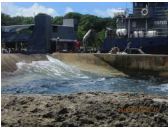
Figure 42 Wave run up and over topping
