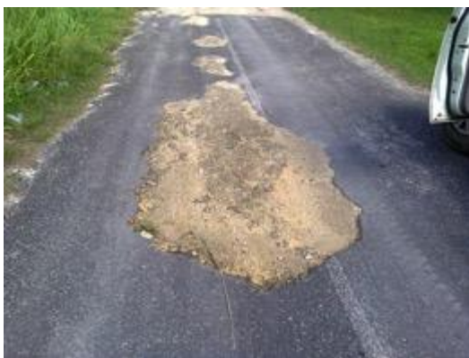
Figure 14 Pavement and shoulder breaking up on Efate and Ambae roads
