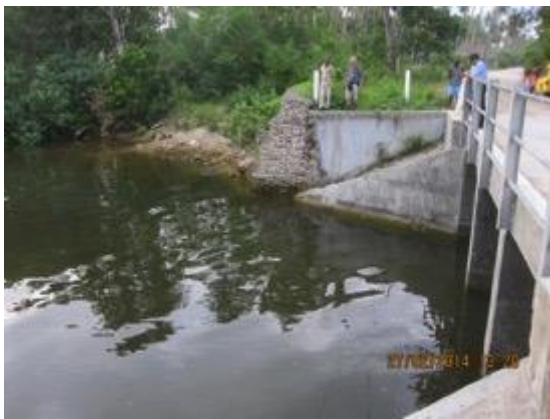
Figure 34 Gabions used in water crossings (Malakula)
