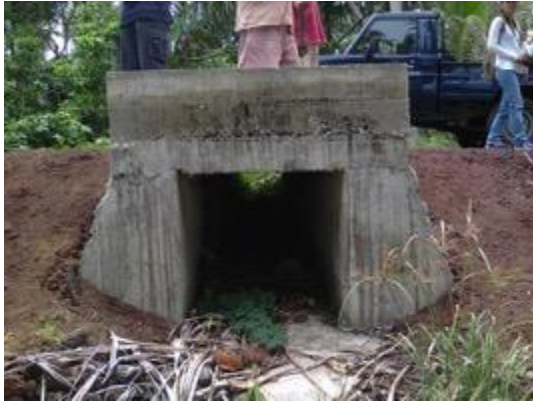
Figure 24 Box culvert from concrete and pipe culvert from corrugated metal sheeting on Malakula
