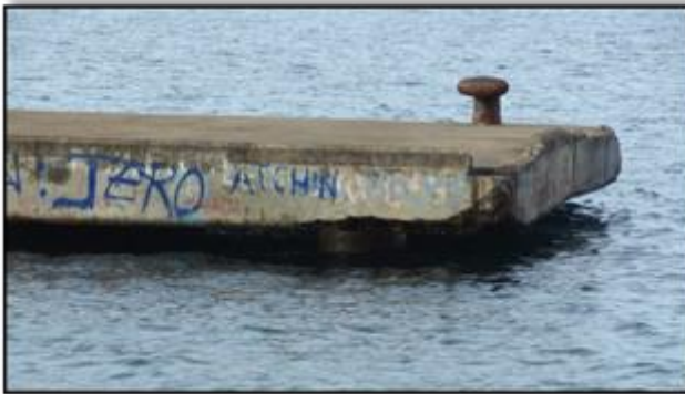
Figure 43 Wharf with low free board at high tide
