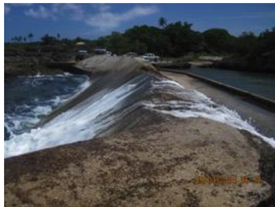
Figure 42 Wave run up and over topping
