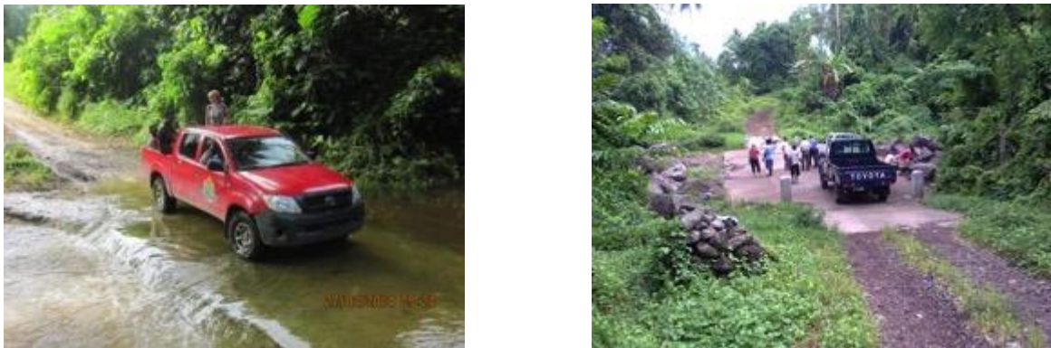
Figure 36 Low Level Crossing with flow and drift guideposts
