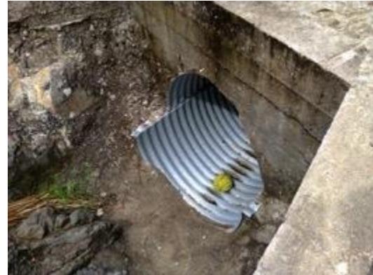
Figure 24 Box culvert from concrete and pipe culvert from corrugated metal sheeting on Malakula
