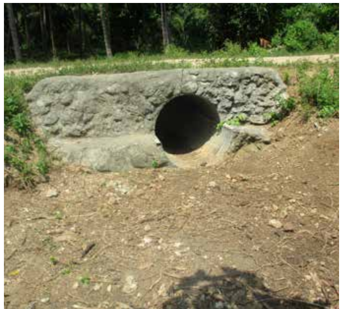
Cleared culvert, South Road, Santo
