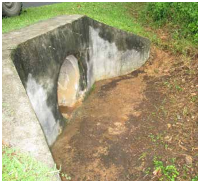
Cleared culvert, South East Coast Road, Santo
