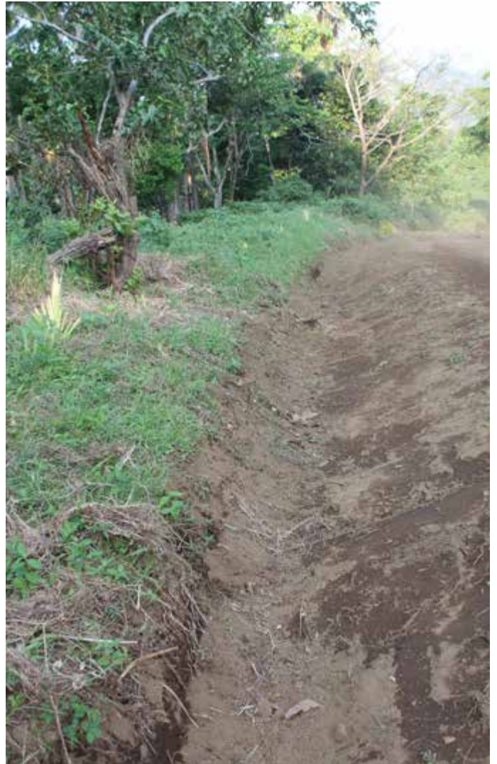
Cleared side drain, North Ambae Road
