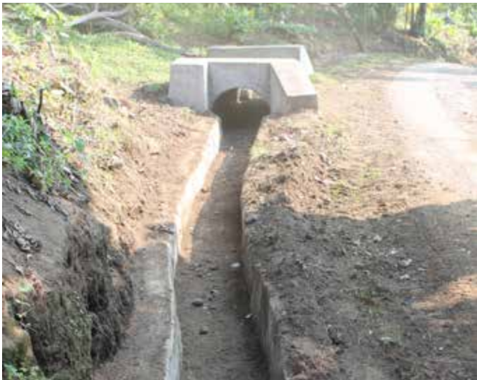
Cleared side drain, East Ambae Road
