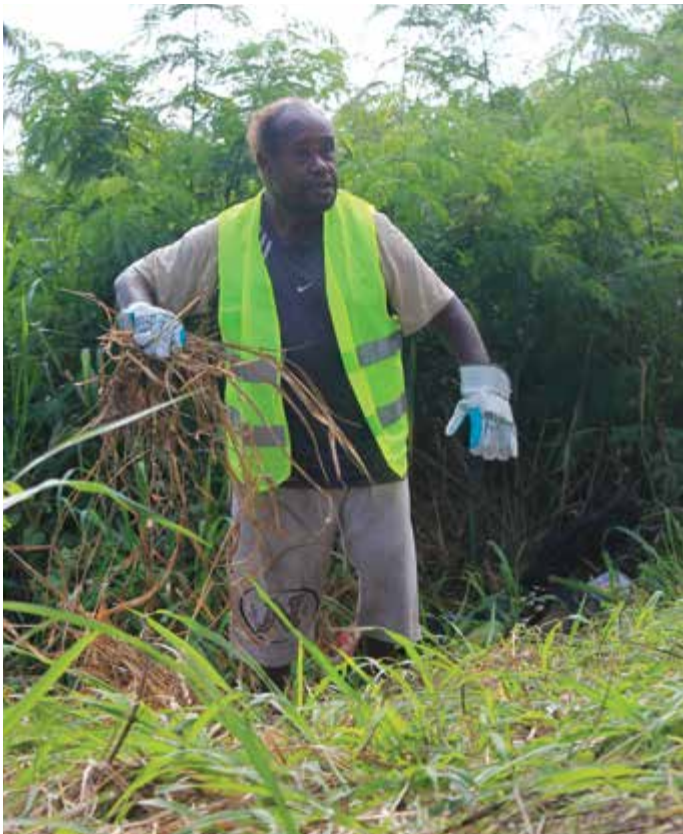
Kaltong Jimmy hemi kat problem blong no save toktok gud be hemi wok tu olsem wan kontrakta long Efate Rinf Rod.
