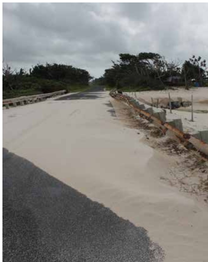
Sand blown over road at Dry Creek, Eton beach, Efate Ring Road
