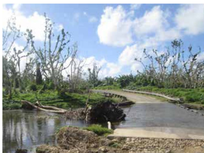
Neilep Bridge, Efate Ring Road
